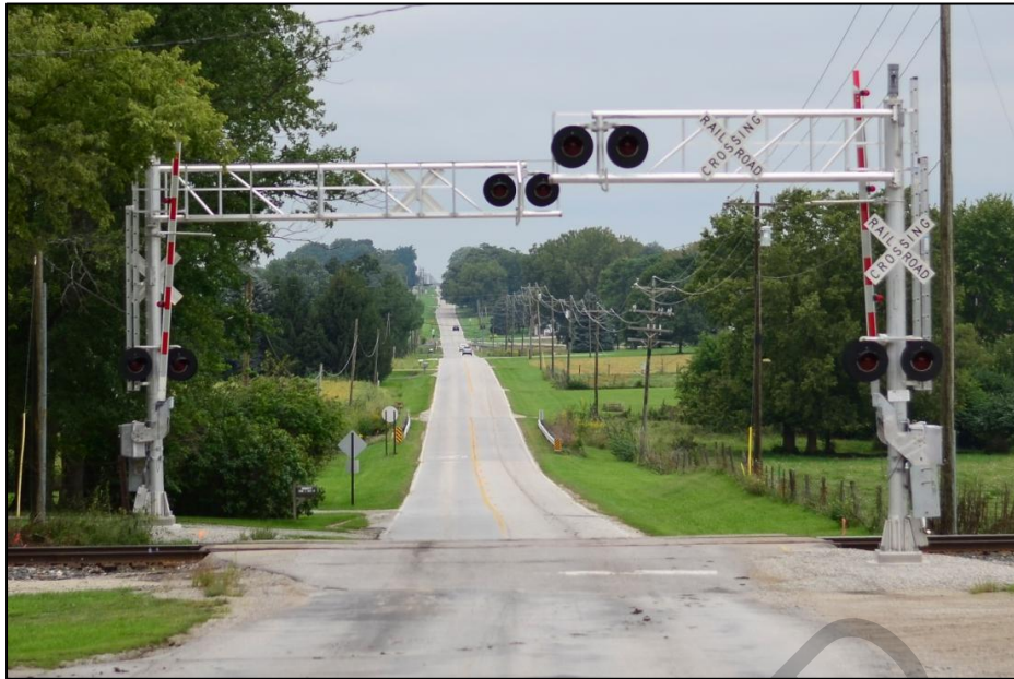
Exhibit 3 Typical Crossing with Active (Train-Activated) Devices
